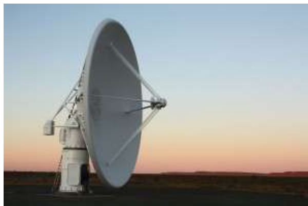
A composite dish is lighter and quicker to build than a traditional dish (click to enlarge)
