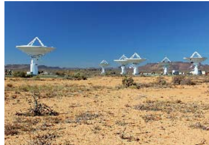
ABOVE: A radio telescope has to be built in a dry area because too much moisture in the atmosphere can absorb the radio waves it detects. This is why the arid Karoo is an ideal place to build the SKA.
