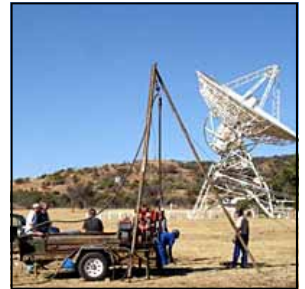
Core drilling at KAT prototype site at HartRAO.
