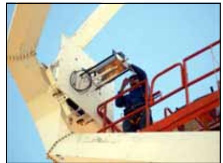
Fig 2: The 1.42 GHz (left) receiver fitted on the dish. On the right Pieter Stronkhorst is busy fitting the 12 GHz receiver.
