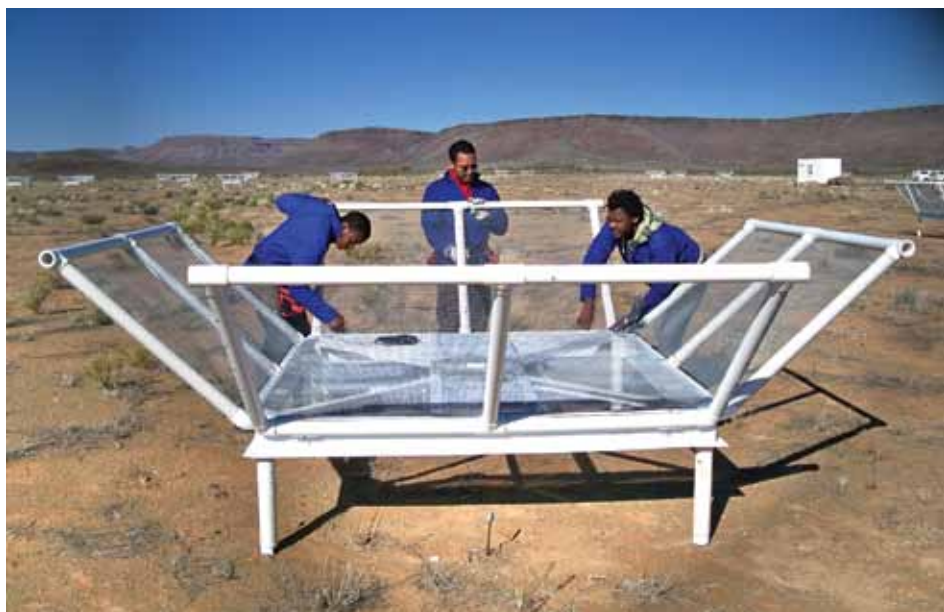
Intern technicians from the Hartebeesthoek Radio Astronomy Observatory helped to install the new PAPER antennas – they are (litr) Monde Manzini, Raphael van Rensburg and Khulekhani Zulu.
