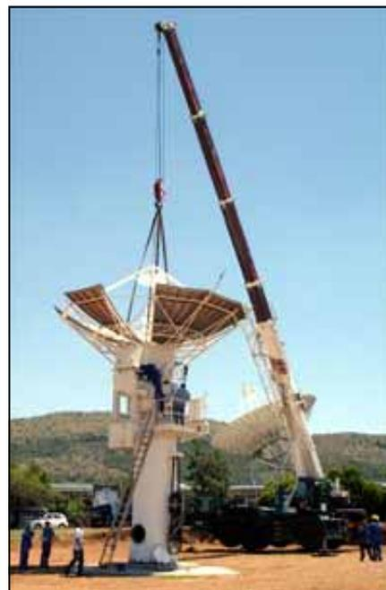
Delivery of the 7.2 m C-BASS dish at HartRAO on 14 February 2007. The C-Band All Sky Survey (C-BASS), will map the whole sky in temperature and polarization at 5GHz.
