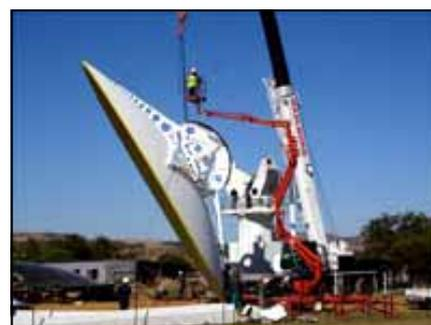
Lifting the dish onto the pedestal; followed by installation of the feed support legs
