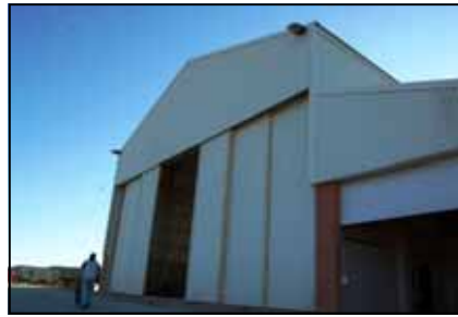
MeerKAT dish construction shed
