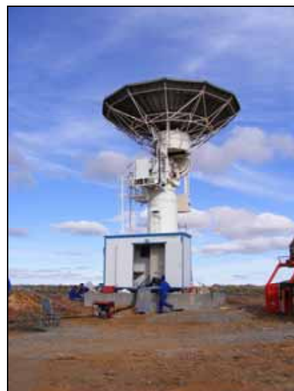
Completed C-BASS antenna with control and instrumentation container in the front
