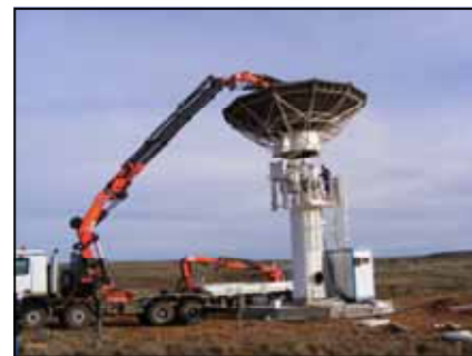
C-BASS dish being lifted into position
